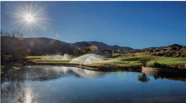
Remodeled lake with stone walls
